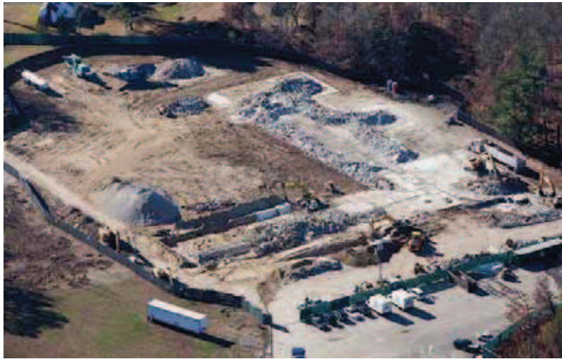
Figure 38. Demolition of Sandy Hook Elementary nearing completion (November 13, 2013)
